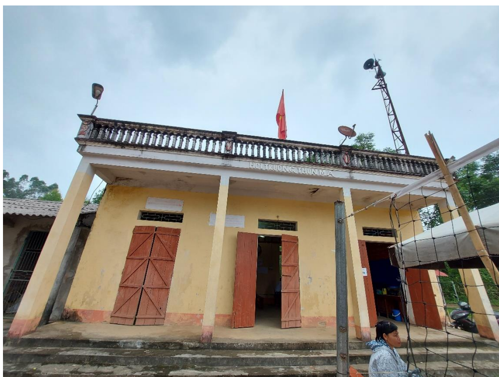
Picture 7. CSV's loudspeaker system in Vinh Kien
